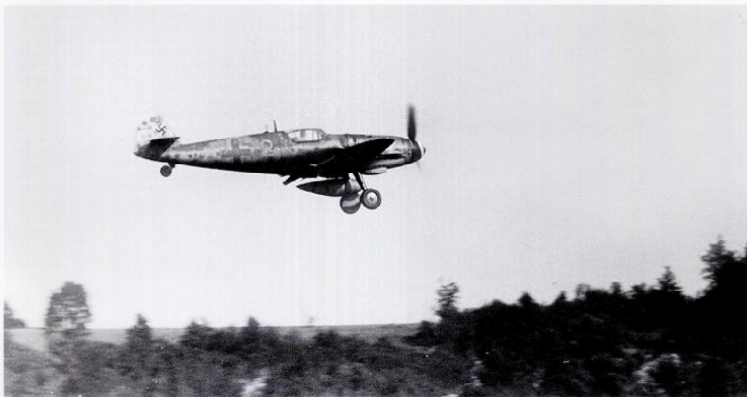
ABOVE: 'Yellow 2', a heavily exhaust-stained Bf 109 G-14 of 9./JG 1, landing at La Fère in July 1944. The aircraft has an Erla canopy and tall tail unit, and clearly visible on the fin is the W.Nr. 413553.
